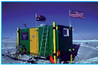
The AFOS building: the 'warm room'
